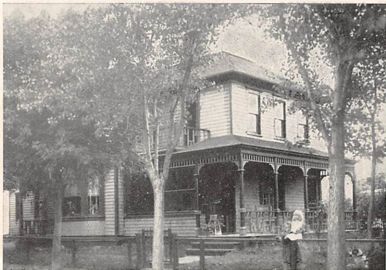
Residence of Geo. K. McEwan Corner of Fifth Street and Harris Avenue
